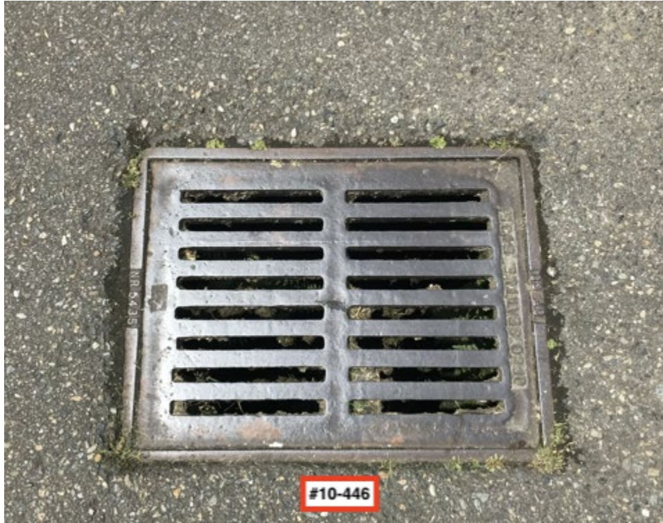
Close up of catch basin #10-446.
