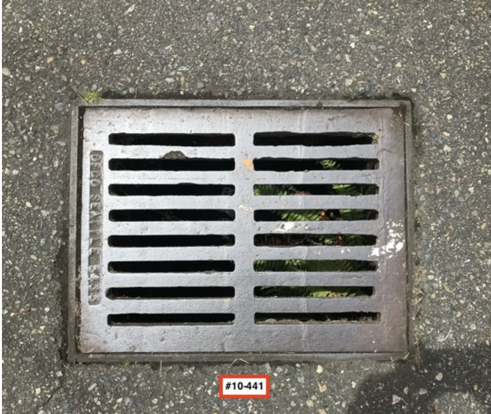
Close up of catch basin #10-441.
