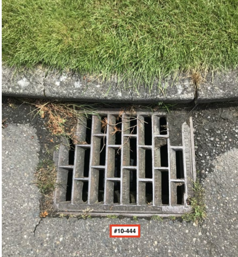
Close up of catch basin #10-444.
