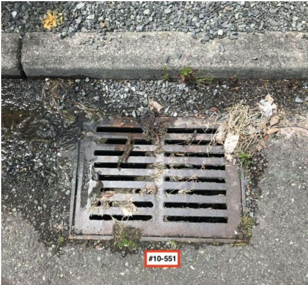
Close up of catch basin #10-551.
