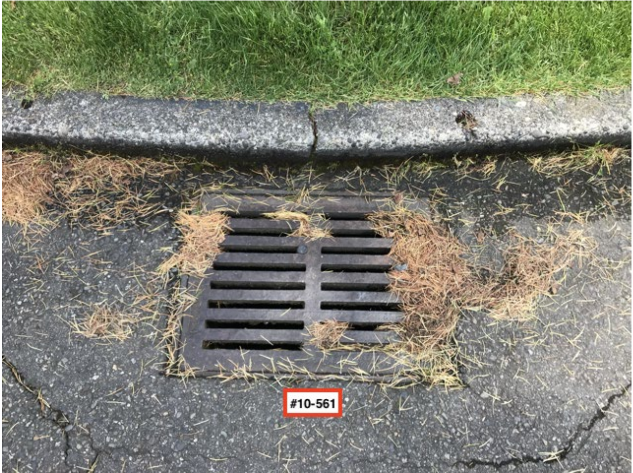
Close up of catch basin #10-561.
