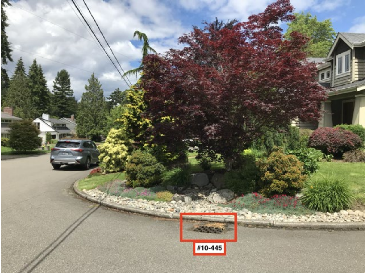
Facing N (downstream) at SE 37th St and 77th Ave SE, catch basin #10-445 in foreground.
