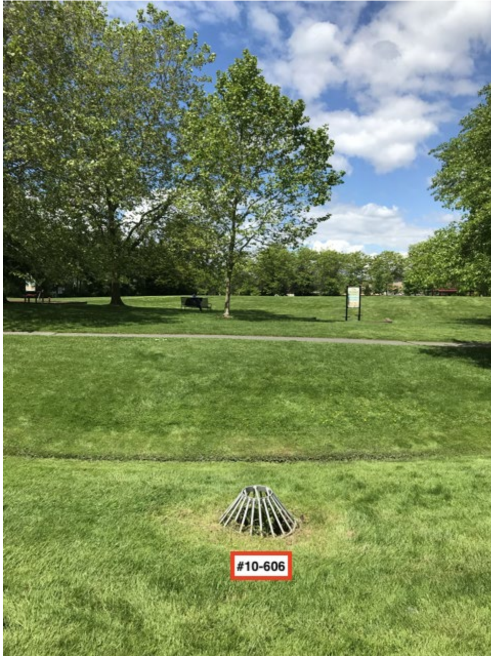
Facing N, with catch basin #10-606 in foreground.
