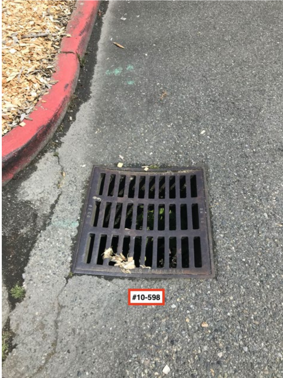
Close up of catch basin #10-598.
