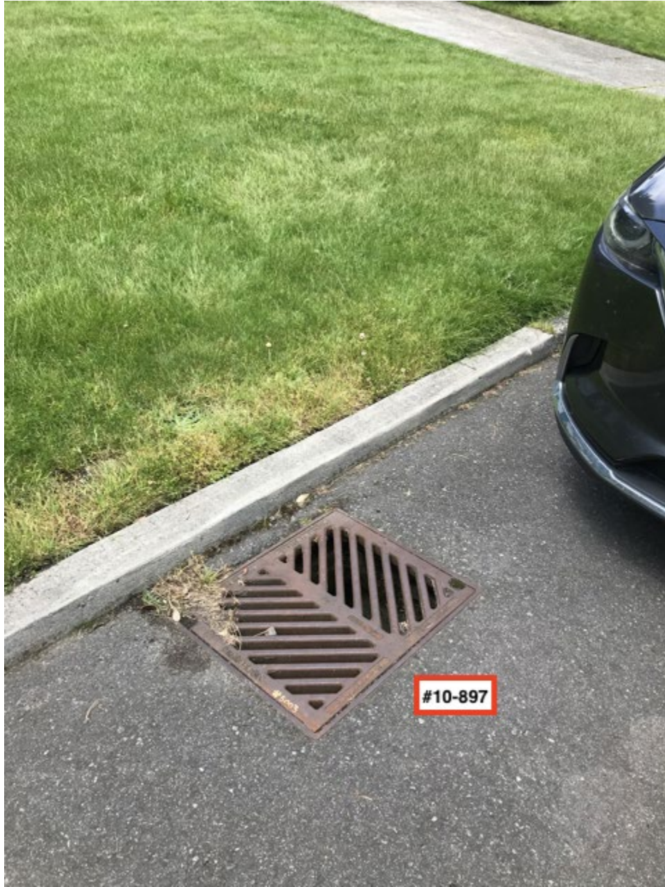
Facing NW on 77th Ave SE, catch basin #10-897.
