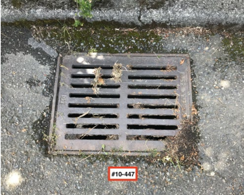
Close up of catch basin #10-447.
