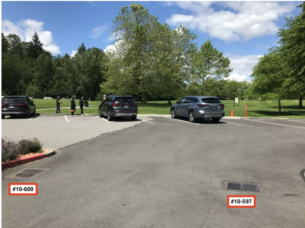
Facing N, catch basins #10-597 (on right) and #10-600 (on left) in Mercerdale Park parking lot off SE 34th St.
