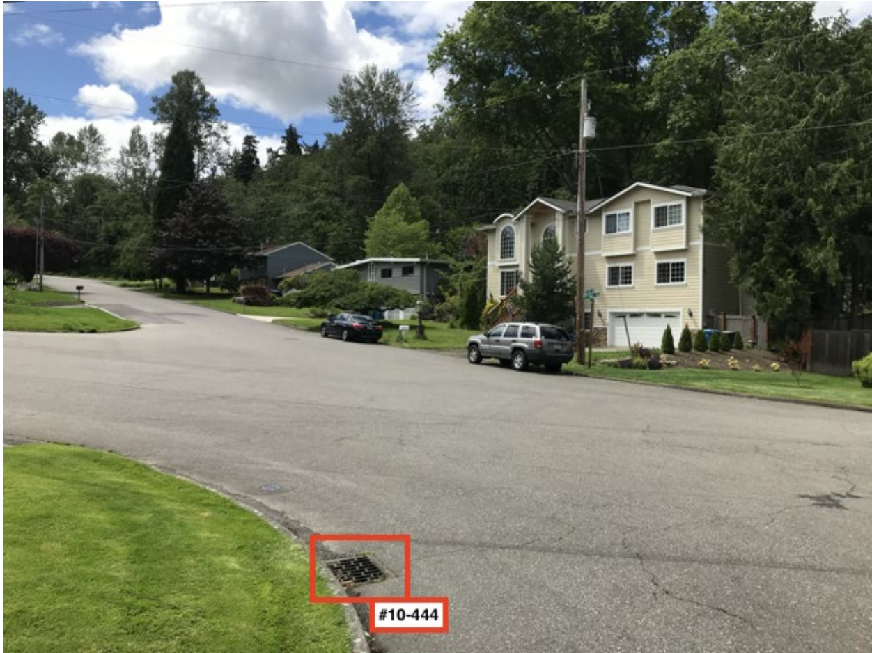
Facing W at SE 37th St and 77th Ave SE, catch basin #10-444 in foreground.
